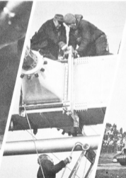
Mounting and installation of the 500 kW short wave antenna LP 501
